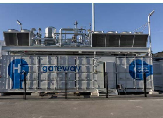
Hydrogen production unit in Vão
