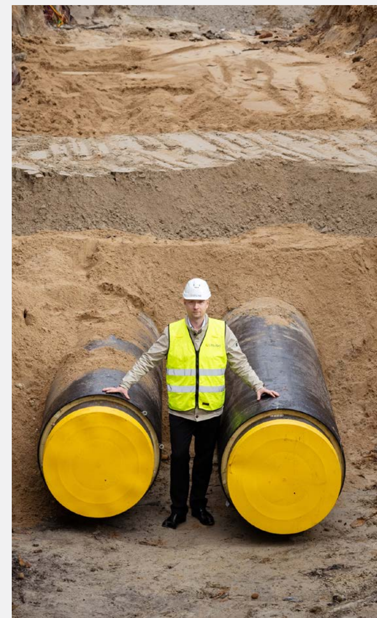
District cooling network construction works in Tallinn
